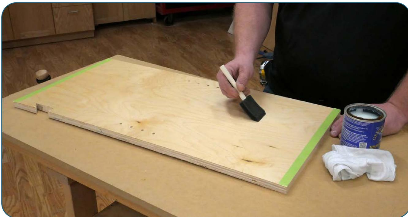
Apply two coats of water-based polyurethane to all surfaces. Lightly sand between coats.
