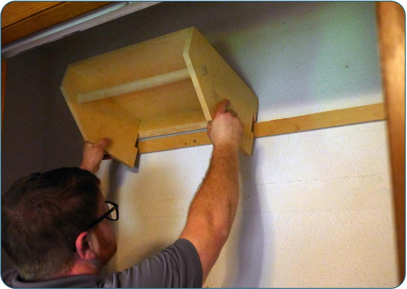
Attach the French cleat rail to the back wall of the closet. Drive 2-1/2" screws through the rail and into wall studs. Hang the cabinet components on the rail and secure the cabinets each other with 1-1/4" screws.
