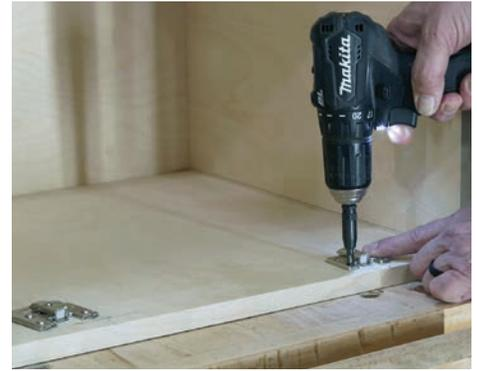
9) With a Vix bit in a drill driver, drill the screw holes for the hinge plate, using the divots to accurately locate the holes.
