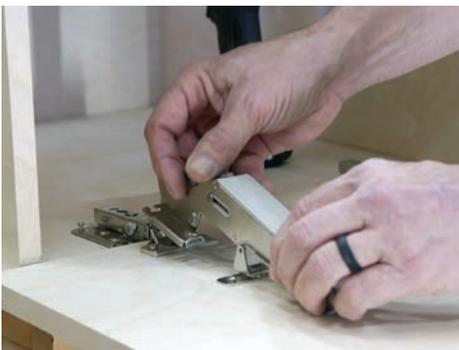
13) Remove the forward two screws on the lid stay hinge plate. Loosen the rear two screws. Slide the lid stay onto the lid stay plate.
