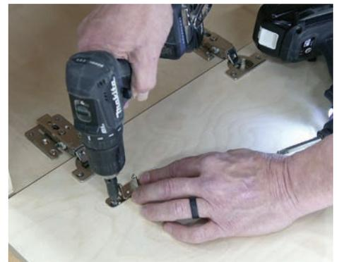
12) Bore the holes for the Aileron lid stay plate. Mount the lid stay plate.
